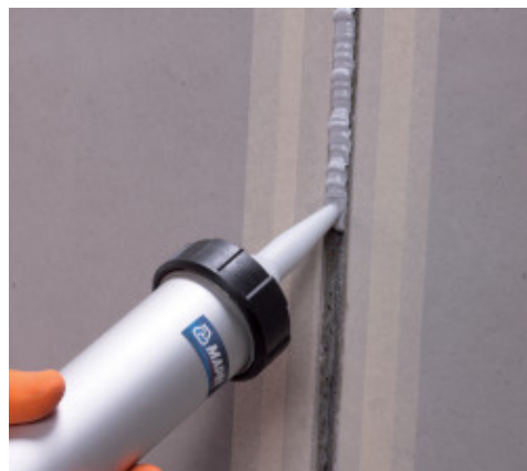
Application de Mapeflex PU40
